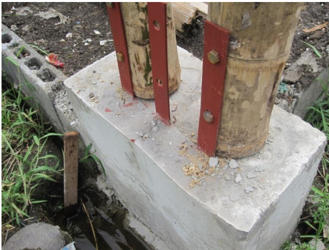
Fig. 6. Column and Foundation Connection.
