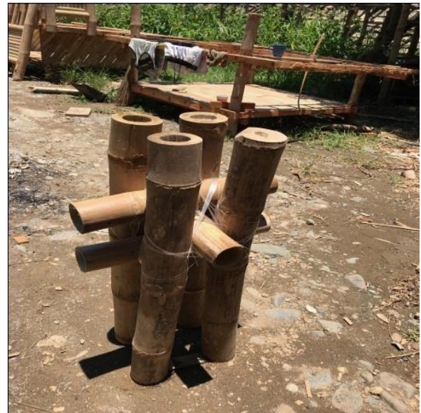
Fig. 4. Column and Beam Connection.
