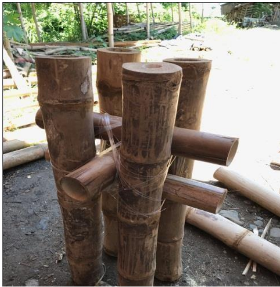
Fig. 5. Column and Roof Connection.
